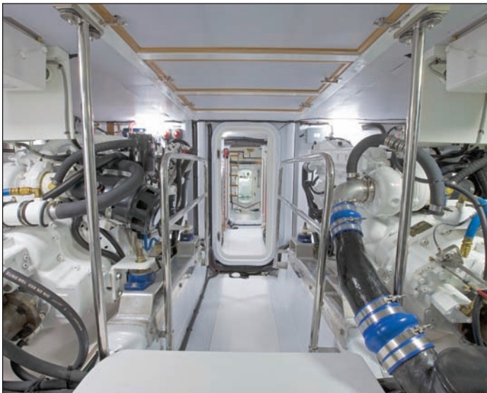
Five watertight doors separate the lazarette from the bow thruster.
