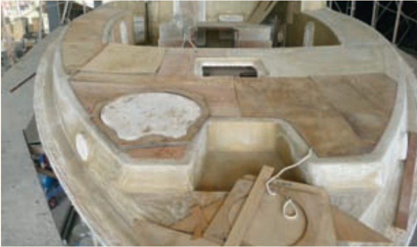
Structures are reinforced with fiberglass stiffeners.
