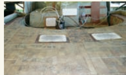
All decks are cored and vacuum bagged.
