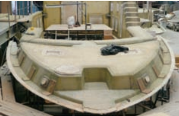
Backing plates under the cap rail will hold stanchion hardware.
